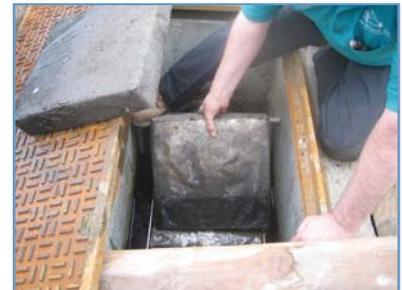
Smart Sponge Vaults can also be designed for spill containment and aid in meeting Spill Prevention, Control, and Countermeasure (SPCC) requirements. The Smart Sponge media will completely encapsulate or prohibit the conveyance of the designed spill volume, so there is little risk, if any, of hydrocarbons being discharged off site, even for large spills.
