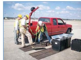
The Ultra Urban Filter Drain Insert Series offers the same filtration characteristics of the CO series for stormwater filtration of hydrocarbons, trash and sediment. The unique micro porosity of Smart Sponge allows a hydraulic flow rate between 200 and 500 gallons per minute based on the filter size and has proven effective in removing more than 80% of hydrocarbons.
