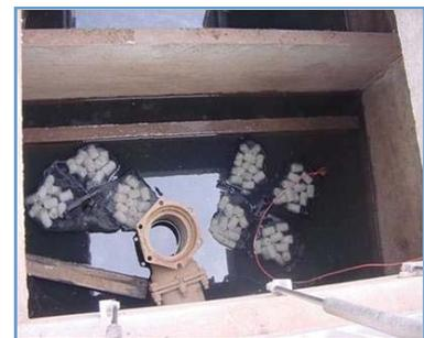
the oil within the Smart Sponge rather than pumping away oily water with oil concentrations of 1000ppm. By extending these test numbers to all 38 OWIs on site at RAF Coningsby the potential savings was calculated as £33,948, approximately \$50,000 US (64%), and 1,258.6 tons of waste (99.9%).
